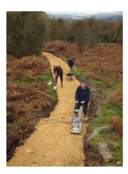
Major path restoration work has been completed on Ilkley Moor. Starting from the Wooden Bridge at Backstone Beck, new steps have been made on the first steep part of the path, the sandstone path continues for 350 metres to the lower Tarn.
